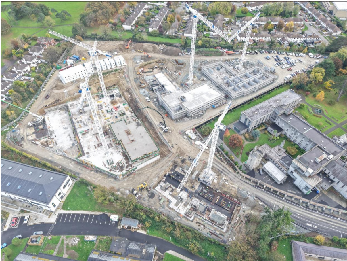
Figure 1 Image of wider site, with blocks A to D currently under construction
